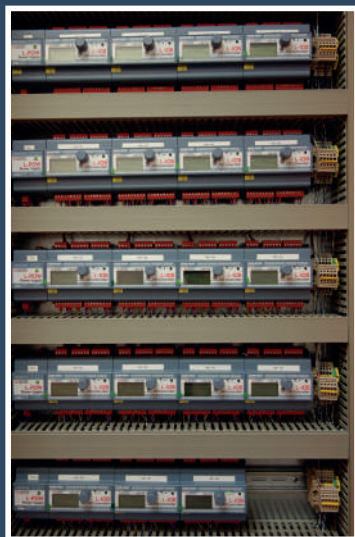
Sub-distributors with L-IOB Modules
